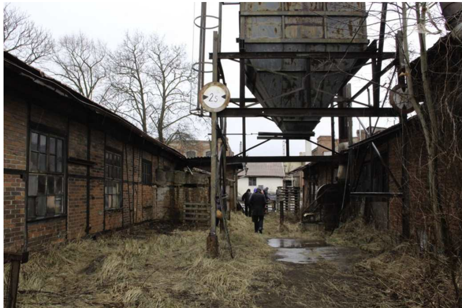
Figure 34. On site at Zbůch: Case Study site
