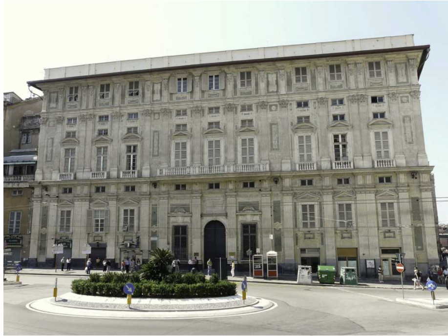
Figure 32. Genoa: Palazzo Belimbau Case Study, the front elevation belies its complexity
