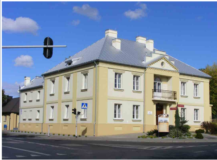
RADOMSKO, Multi-family residential building
